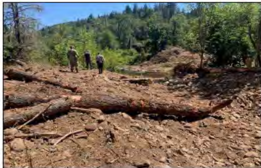
Side channel excavation with large woody debris. Logs donated by BLM and Hancock Timber- salvage from 2018 Miles wildfire that burnt 200+ ac in Elk Creek.
